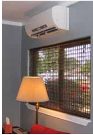
The indoor head of a ductless system sits unobtrusively above the window.
