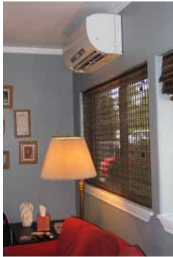
The indoor head of a ductless system sits high on a wall. The outdoor unit is more compact than a typical whole house air conditioner.
