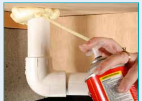
Sealing around plumbing penetrations and caulking & weather-stripping around doors and windows will help keep heat in.
