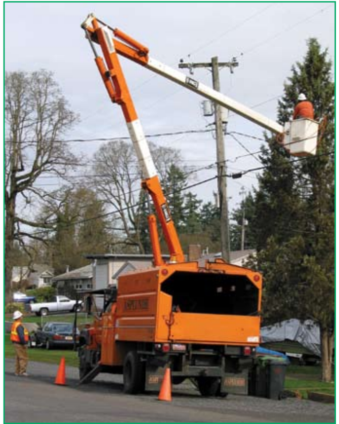
Tree crews work year-round to maintain clearance between PUD power lines and nearby trees and shrubs.
